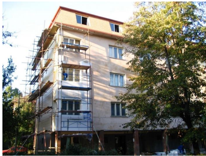
Figure 4. The pilot building under reconstruction
