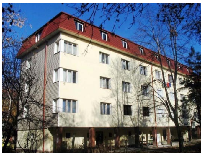
Figure 5. Renovated pilot building
