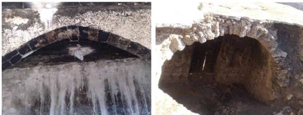
Fig. 3. Structural Arches support the ceilings, the pictures are for house No. 1 Block 1 (right) and house No. 3 Block 3 (left) (Author, 2016)
