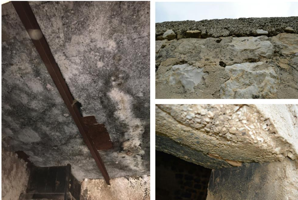
Fig. 2. A ceiling structural system of cement and I beam (Author, 2016)
