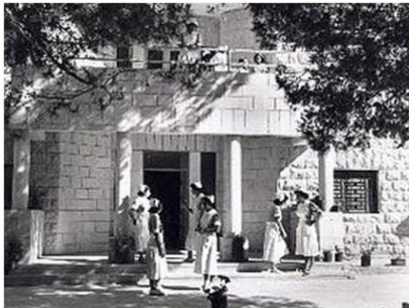
Fig. 6. Baptist Hospital built in 1952, which re-used later as a school for nursing (Source: Denomination Jordanian Baptist Church web site)
