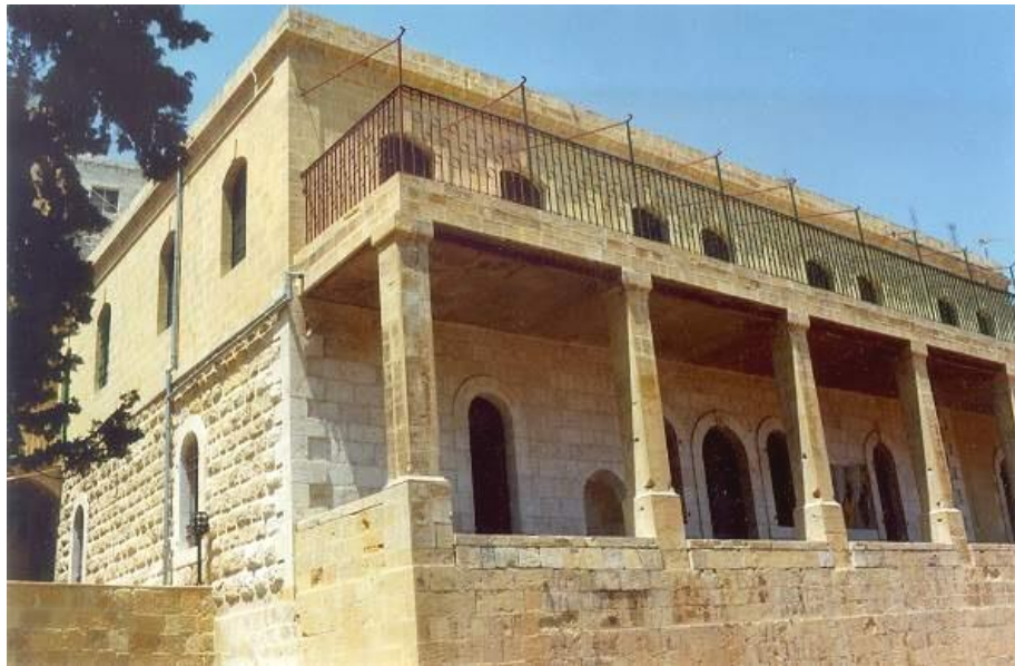
Fig. 1. General view of the Old English Hospital
