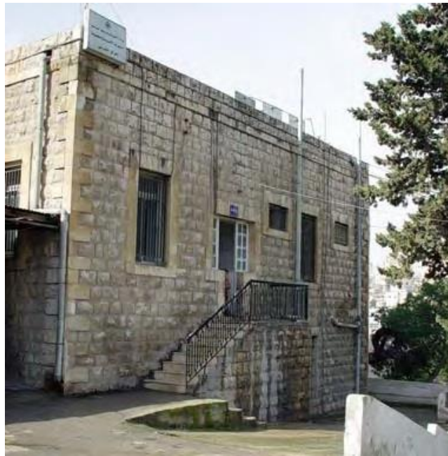
Fig. 3. Front elevation of the English Mission Hospital (Source: Shawash 2003)
