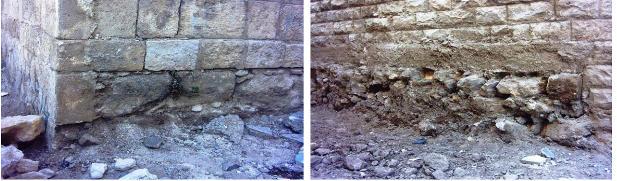
Fig. 5. First maintenance stage
