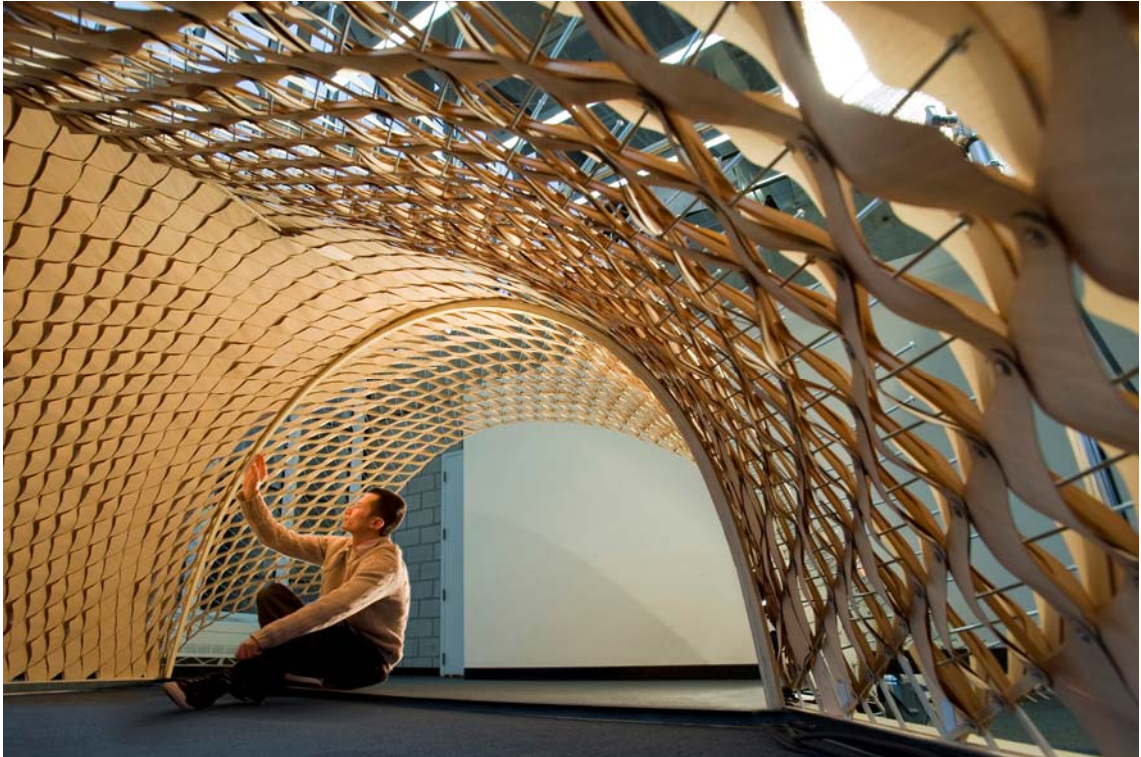
Fig. 5c. Double curved wooden lattice.
